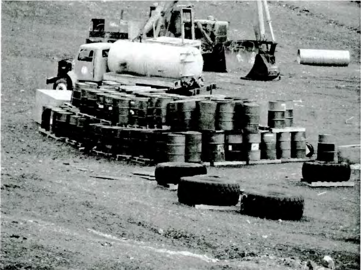
Picture 1 : general view of the hazardous waste storage area, Kangijsujuaq
