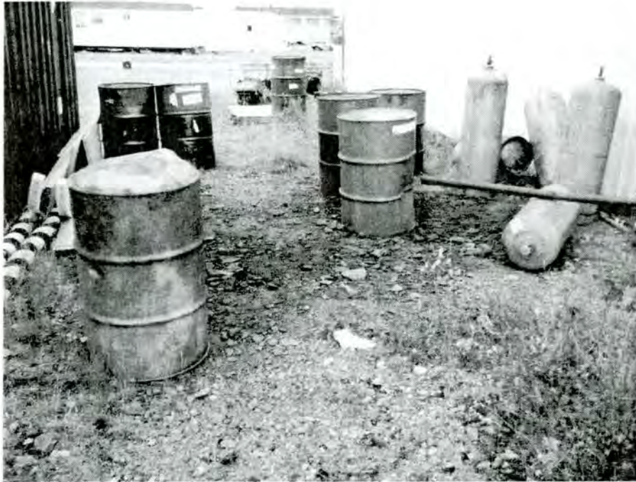
Picture 7 : Barrel and gas cylinder storage area with hydrocarbon stain, Tasiujaq
