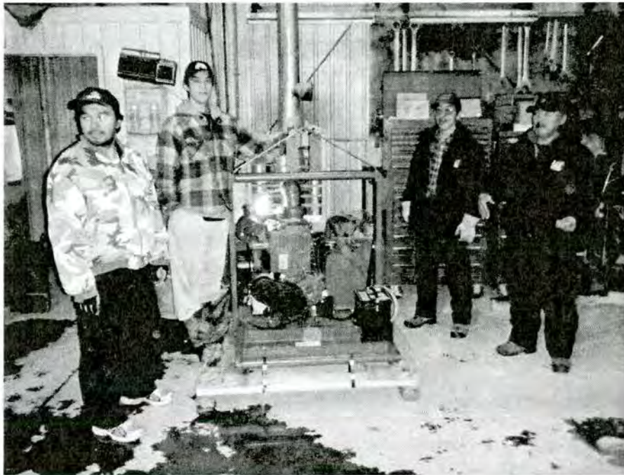
Picture 12 : Waste oil incinerator, Inukjuaq
